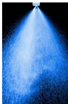
Picture supplied by SE Fire Sprinklers Ltd
